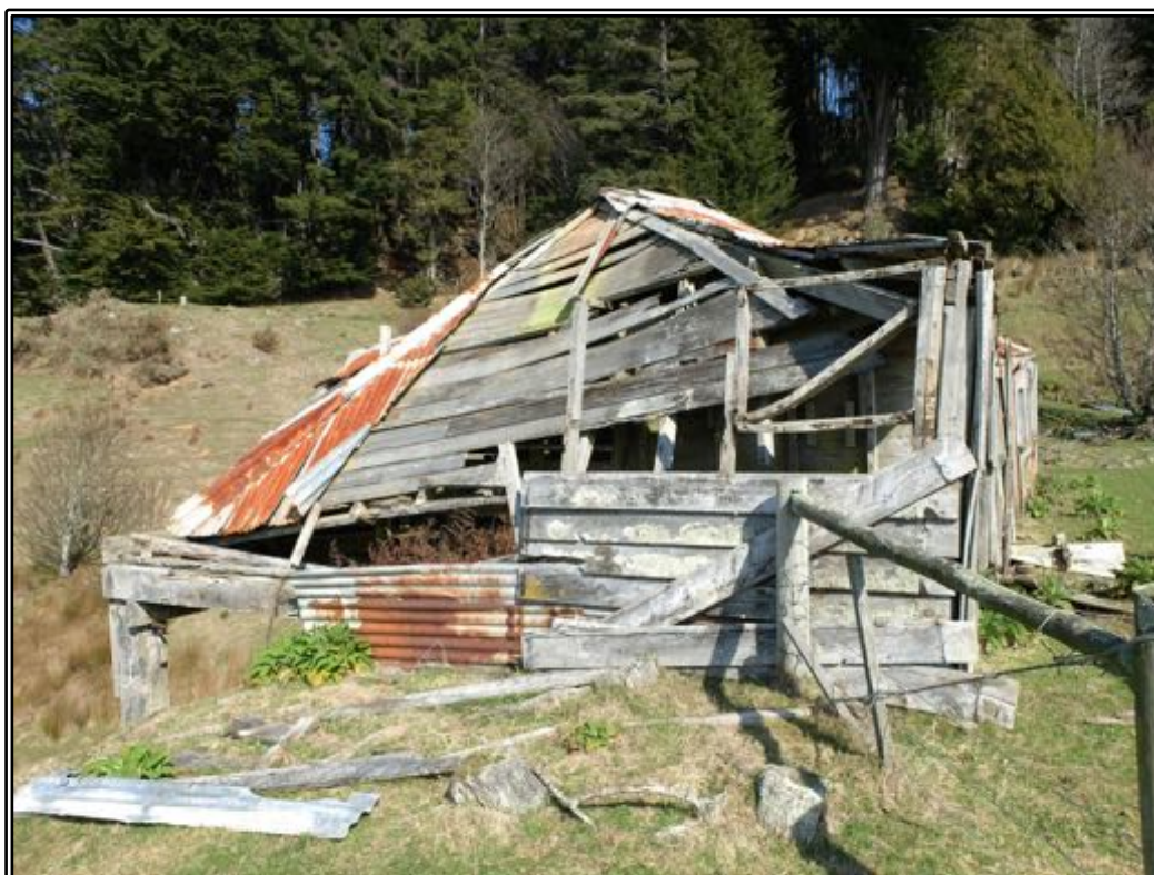
Figure 15 The collapsed east wall, with the collapsed hip roof, in 2017.
