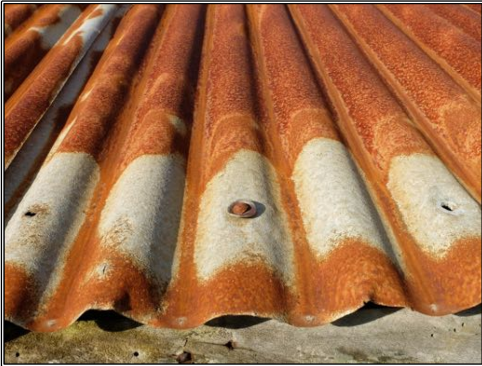
Figure 36 Detail of the corrugated iron roof cladding, showing the lead-washer roofing nails that were used to fix the iron.
