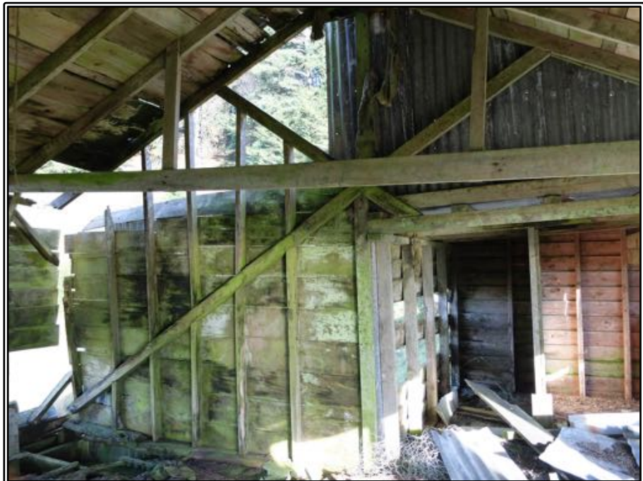
Figure 24 The western end wall showing the cross-brace. This cross-brace is probably the main reason the building was still standing in early 2018. Note the close spacing of the studs in this wall (19 inches centre to centre).
