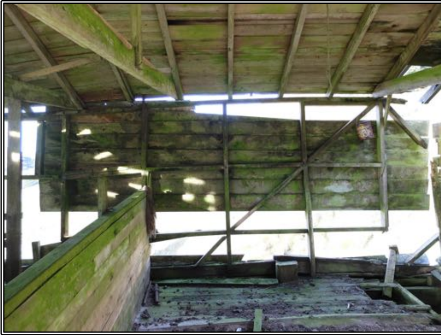
Figure 23 The rear wall framing, of very lightweight conventional construction with widely spaced (37.5 inches centre to centre) studs. By this date (2018) the wall was on the verge of collapse.
