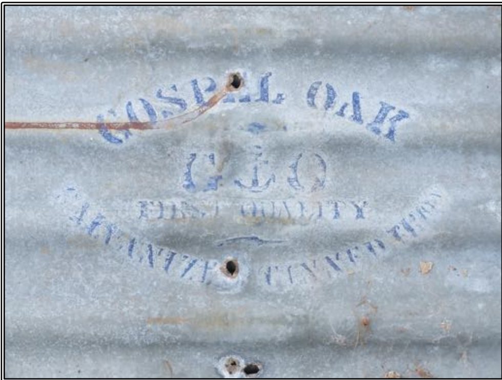
Figure 37 Detail of the maker's mark on one sheet of iron (all sheets inspected were from the same maker); 'Gospel Oak, Best Quality, Galvanized Tinned Iron.'
