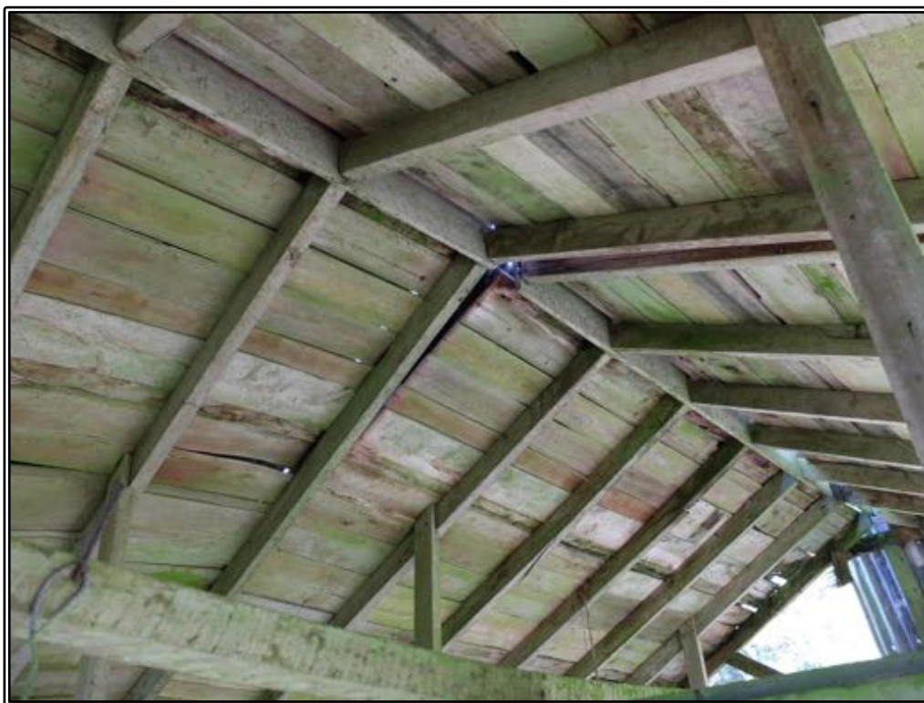
Figure 34 The roof framing, showing the rafters and sarking.
