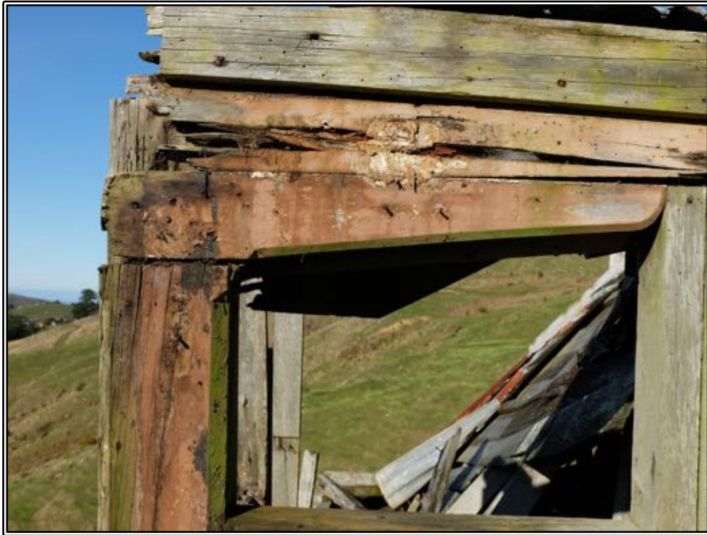
Figure 27 Detail of the easternmost corbel, which had been cut off when the structure was shortened.
