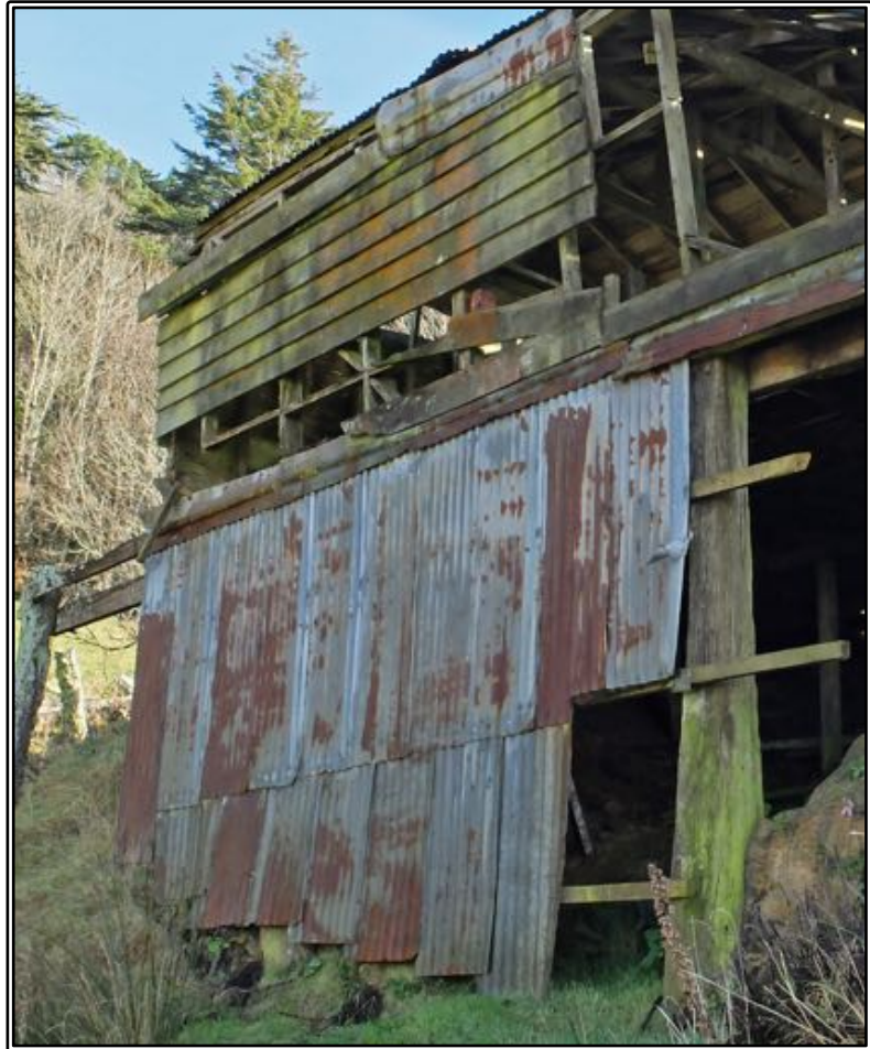
Figure 33 A view of the rear of the building, showing the corrugated iron cladding covering the sub-floor area, and the weatherboards on the wall of the building.
