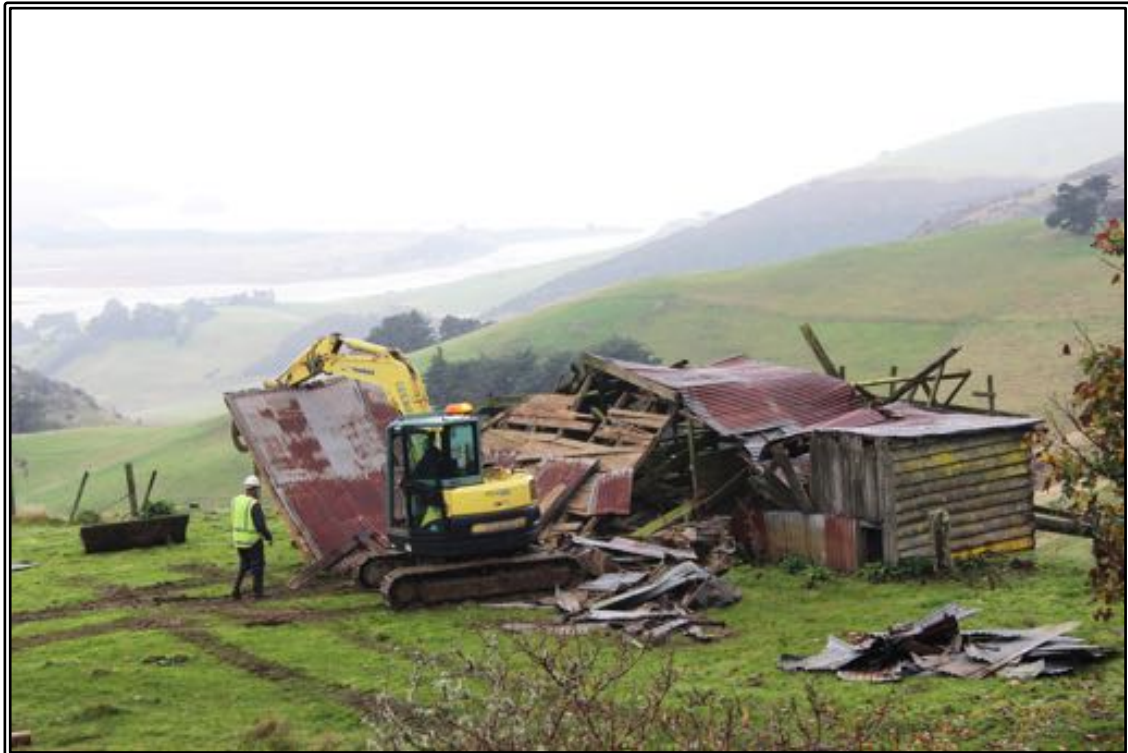
Figure 45 Lifting the roof off the building (Neville Peat).
