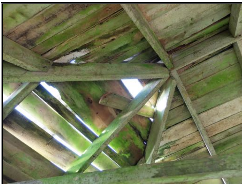
Figure 35 Detail of the ridge structure at the hipped end of the roof.
