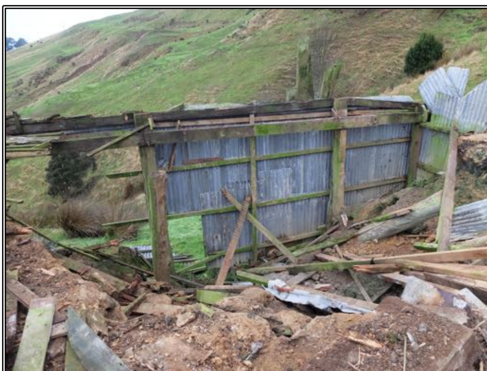
Figure 47 The rear support structure exposed after the removal of the floor.
