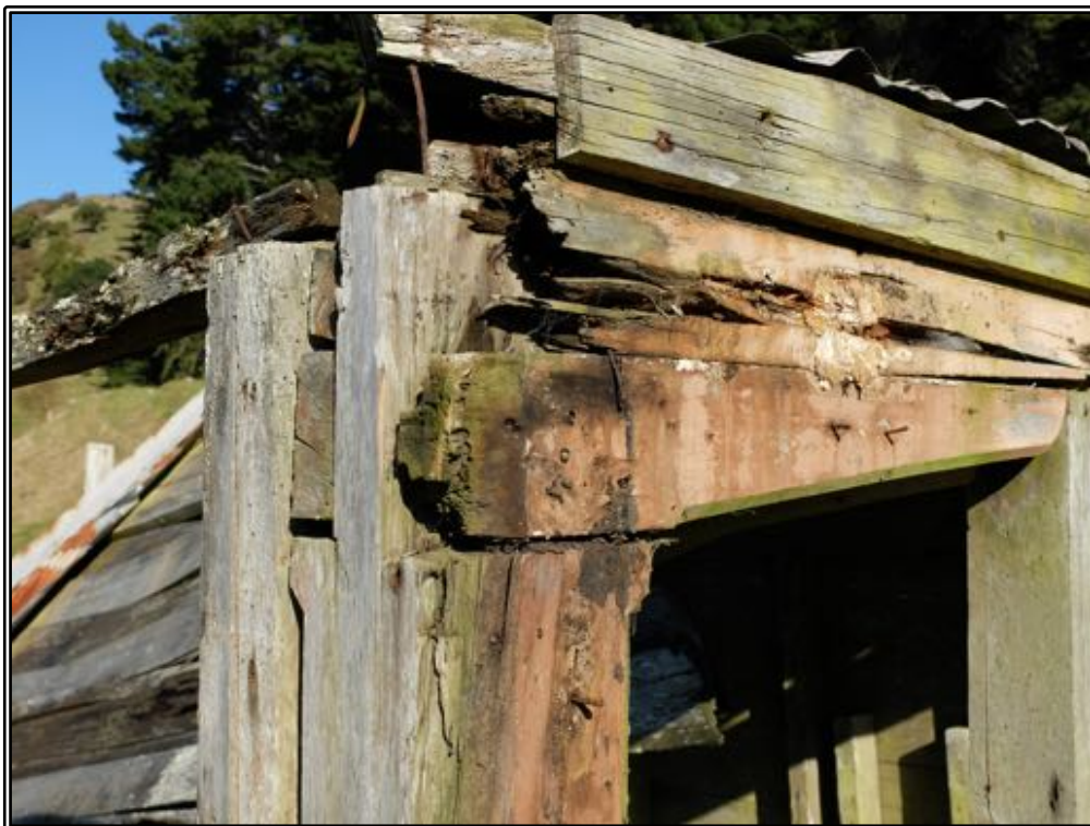
Figure 28 Another detail of the easternmost corbel, with the tenon on the end of the post exposed where the corbel had been cut through. Note that the tenon extended through both the corbel and the plate.
