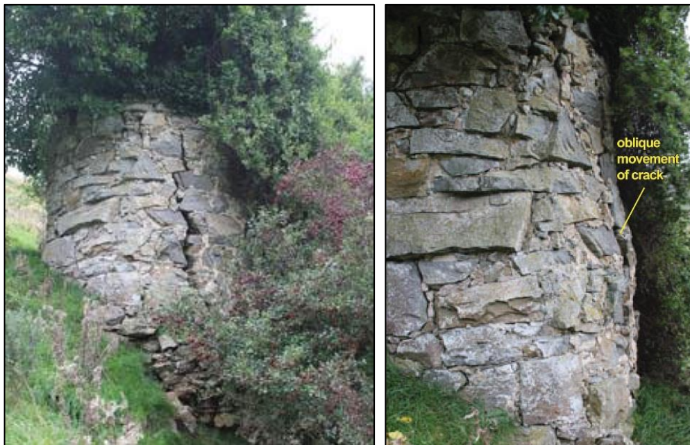
Figure 14. Large crack in the south eastern face of the charging bowl, looking north west (left); a view from the south of the drum exhibiting oblique movement of the crack (right).
