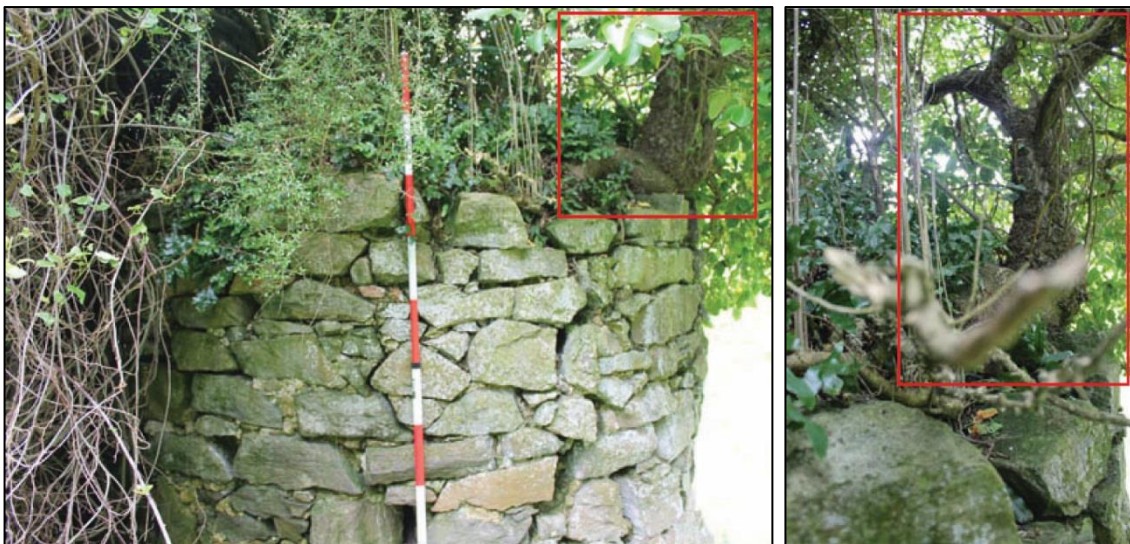
Figure 10. Tree growing out of charging bowl (outlined in red): looking east. Note the crack to the right of the stadia pole (left); looking south-east (right).
