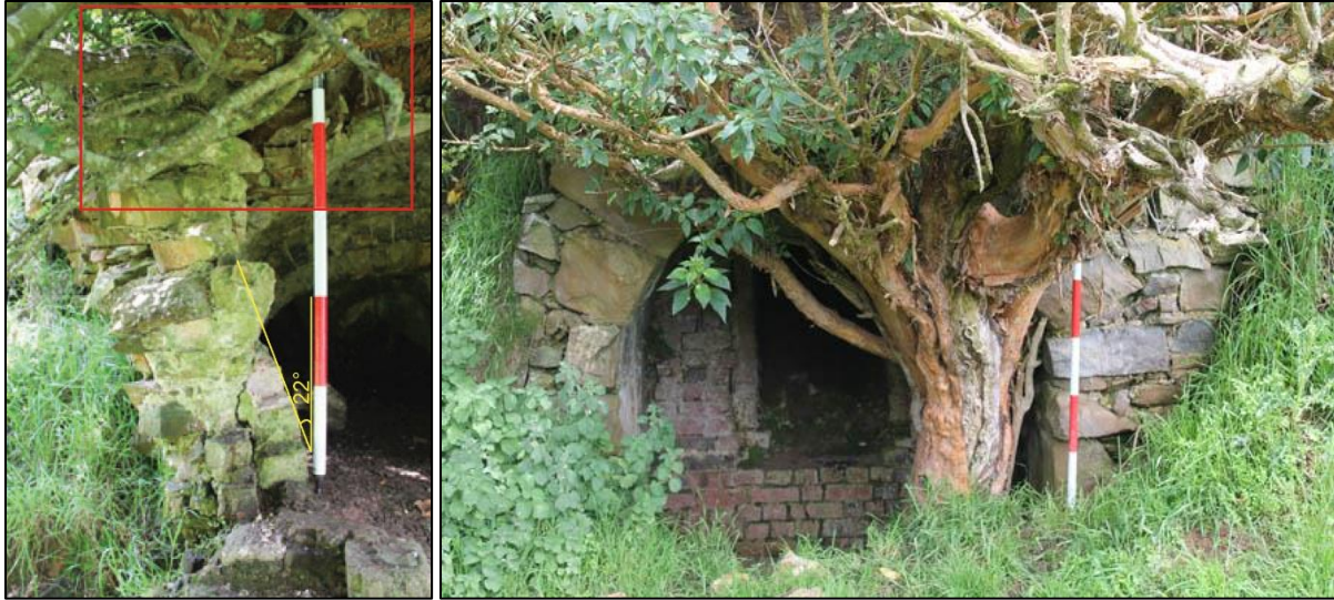
Figure 13. Tree growing out of the firebox roof, looking west (outlined in red: left); Large tree growing in the entryway to the drawing eye chamber, looking west (right).
