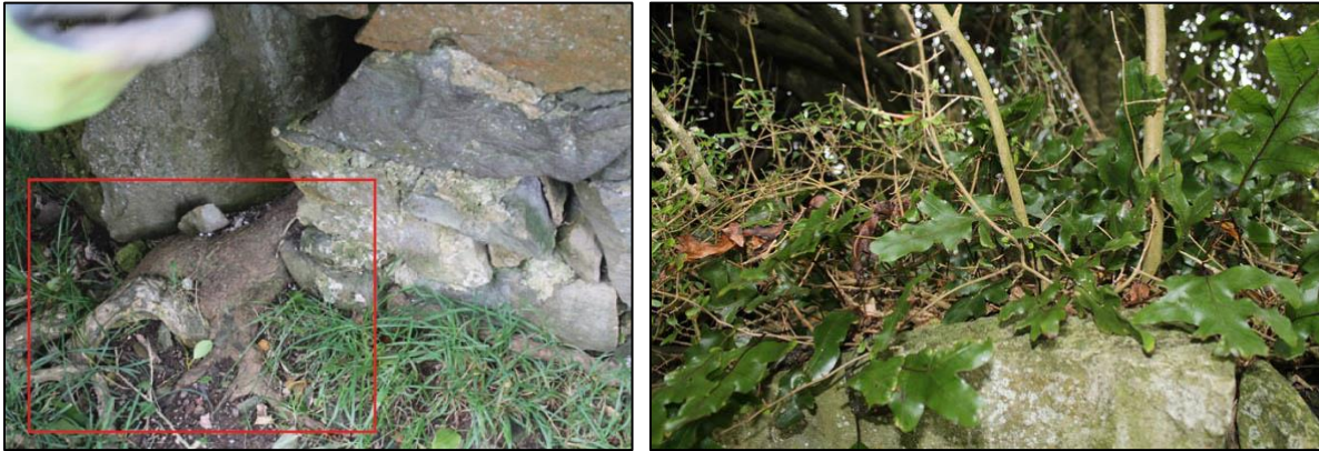
Figure 11. A large tree root (outlined in red) pushing through the masonry and making a large crevice (left); Vegetation growing out of the charging bowl (right).
