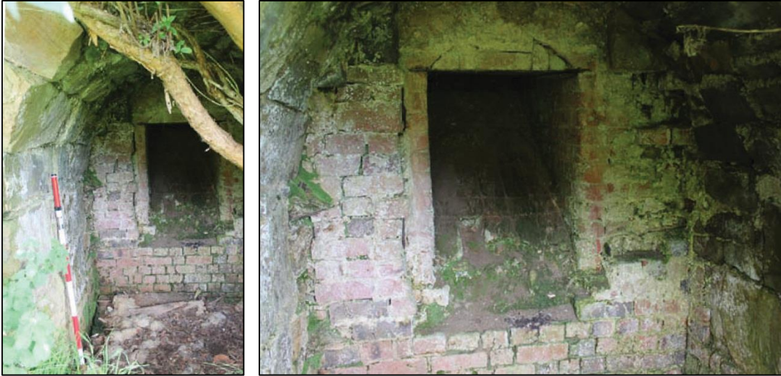
Figure 19. Inner drawing eye compartment: large dressed limestone blocks exhibited in the southern inner wall and the arched roof (left); the drawing eye chute and brick surround (right).
