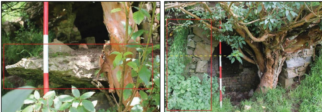
Figure 16. Large concrete slab (outlined in red) which is the platform to the firebox entryway (left); the ground level drops one metre at the junction of the drawing eye entryway stonework (right).
