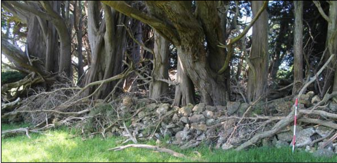
Figure 36. Drywall 4: northern section of the wall with macrocarpa tree branches fallen onto the structure causing massive damage.
