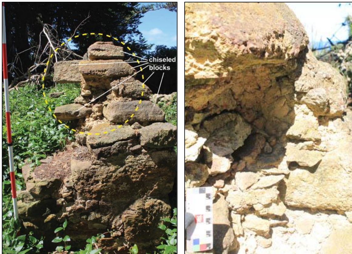
Figure 10. The area within the yellow dashed circle needs to be stabilized, looking east (left); A close-up of the lime/clay mortar used in the wall core, looking south (right).
