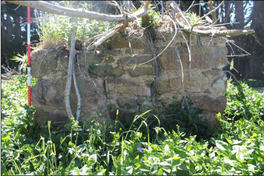
Figure 9. The south-eastern section of the southern wall (looking north) with the dead tree laying over it; note the lime mortar here has resisted weathering.
