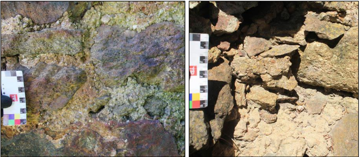
Figure 5. Course lime and tuff aggregate mortar used for the external pointing (left); inner wall core mixture of tuff rubble, clay and lime (right).
