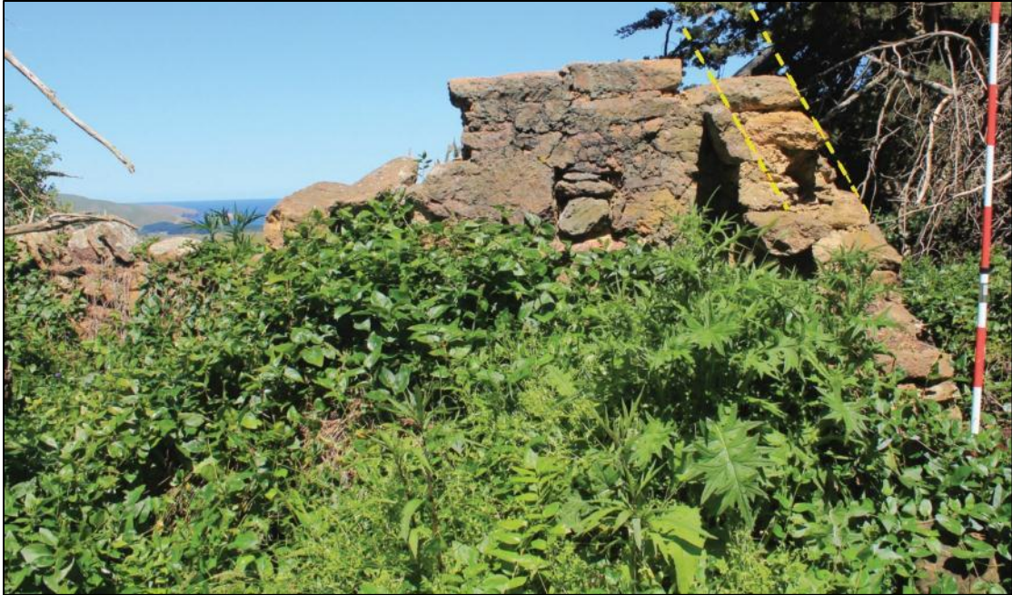
Figure 12. Looking south toward the homestead. The yellow dashed lines in the top right of the image follow the angle (58°) cut into the stone which likely supported a truss.
