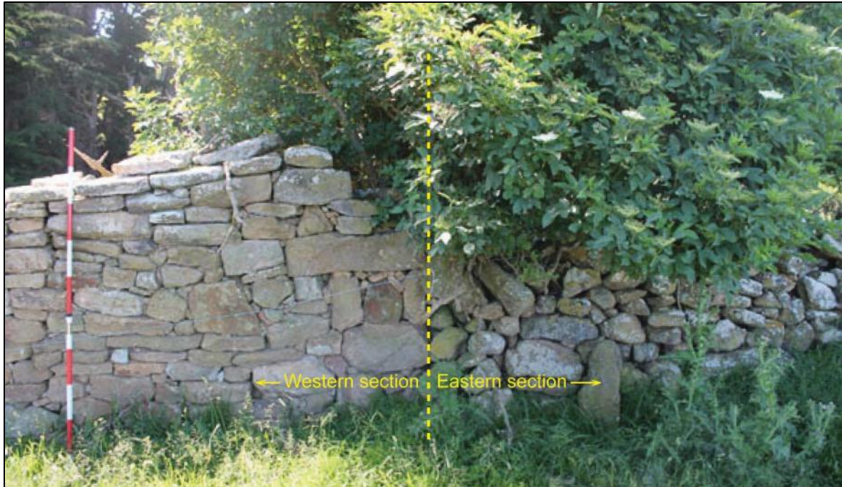
Figure 33. Drywall 3: two separate methods of construction are exhibited either side of the yellow dashed line, looking north.
