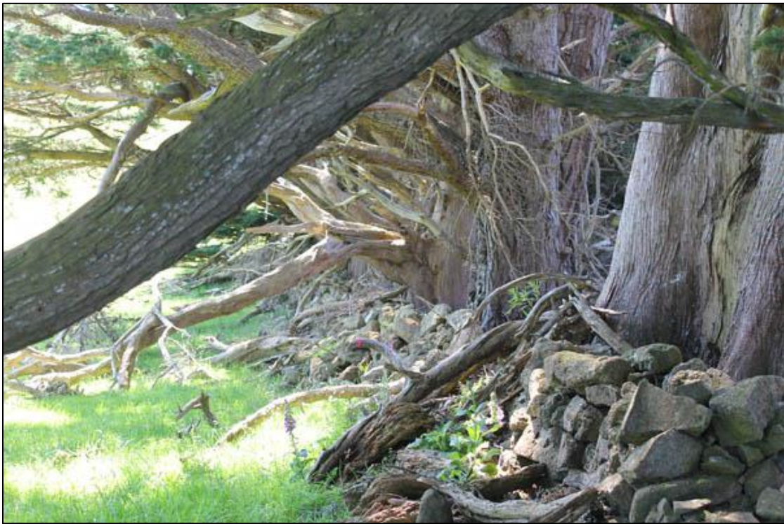
Figure 37. Drywall 3: macrocarpa growth pushing the wall outward.
