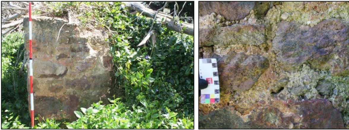
Figure 14. Outer eastern wall, looking west (left); close-up of the masonry in the outer western wall. Note the volcanic tuff used as aggregate in the lime mortar (right).
