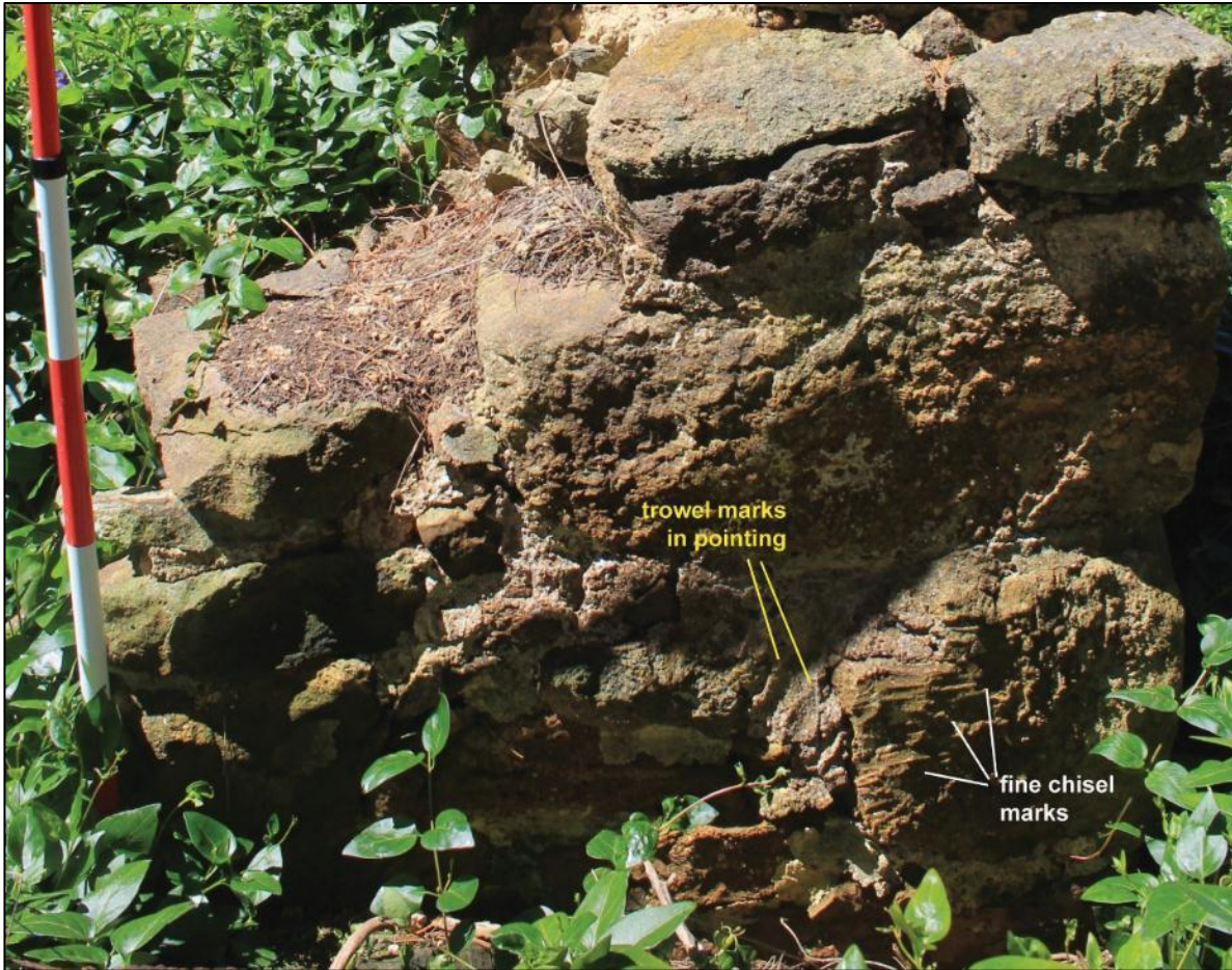
Figure 11. Outer western wall, looking east: trowel marks observed in lime mortar (yellow); fine chisel marks exhibited in the volcanic tuff (white).
