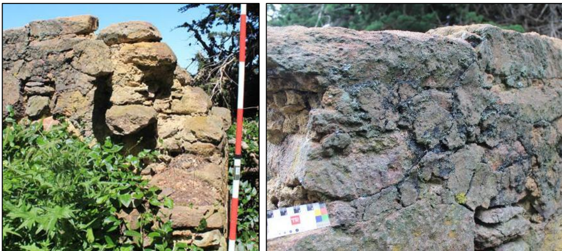
Figure 13. The inner southern wall with large cut blocks protruding northward (left); black pitch/tar used to repoint a section of the inner southern wall (right).
