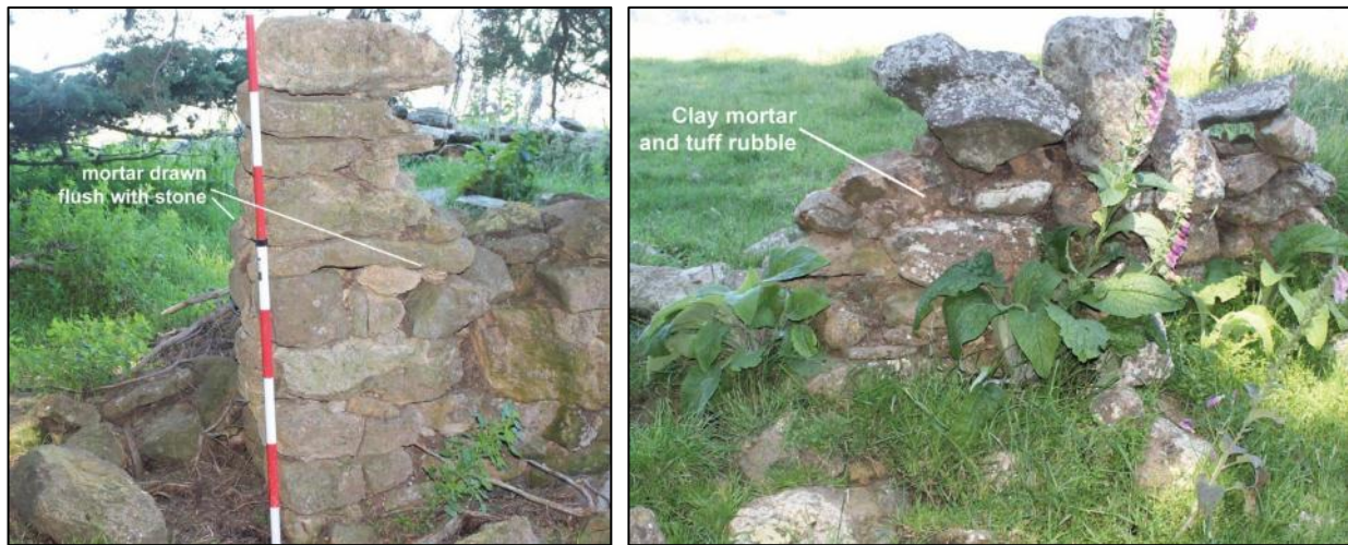
Figure 15. Northern wall end of the cow byre exhibiting remnants lime mortar drawn flush with the stone (left); clay mortar and tuff rubble used in the inner wall.
