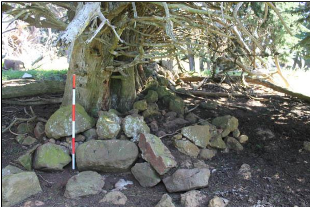
Figure 25. North-western section of Drywall 1 showing the damage caused by macrocarpa growth, looking south-west.
