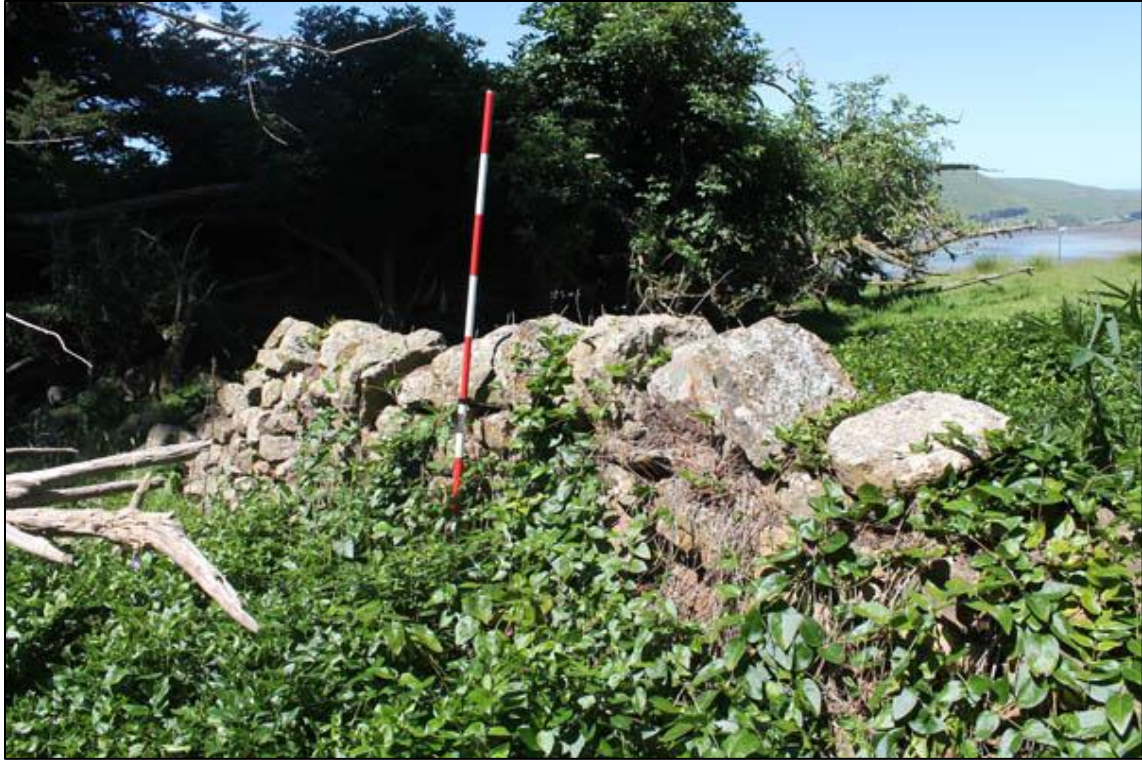
Figure 28. South-eastern section of Drywall1, looking east. Note the coping stones are still capping a large section of this wall.
