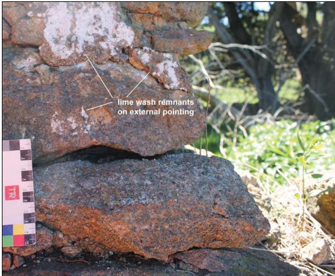
Figure 6. Remnants of a fine coat of lime wash over the external pointing
